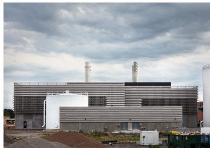
Research and Engineering Center central energy plant. Completed 2019.
